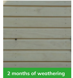
OFFICE SIDING, VROOMSHOOP, THE NETHERLANDS
